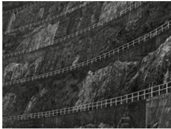
Terraced Rock Wall, Hong Kong – 2015, Photograph
