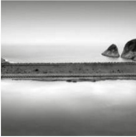
High Island Reservoir Dam, Hong Kong – 2008, Photograph
